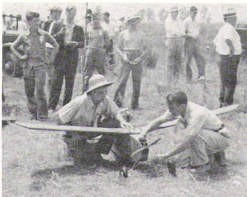
Left: Bill Good built this two-channel transmitter overnight at the local electronics store and then won the meet with it the next day. Center: Bill and Walt prepare the RC Guff for flight. It was fitted for rudder, elevator, and engine control, but only the rudder was used in the 1940 Nats. Right: Bill tuning the receiver with a meter prior to flight—a standard and necessary procedure in the early days. Photo by Al Daraghy.
